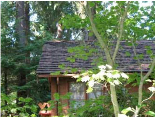
Figure 5-10: Cedar shake roofs are more combustible than composite roofs.
