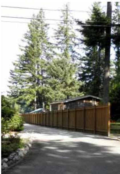
Figure 5-12: Fences connected to houses can spread fire.
