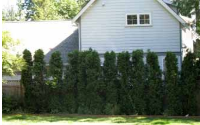
Figure 5-15: Flammable plantings can ignite structures, fences, and poles.
