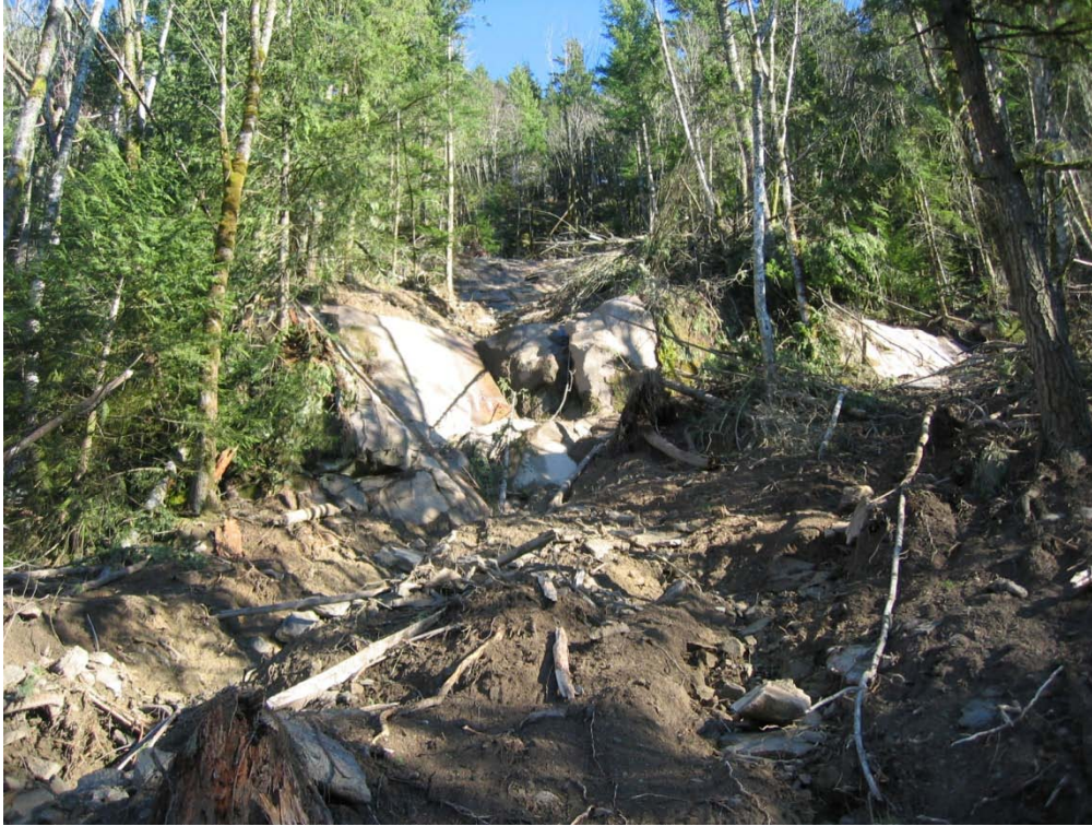
Figure 38 Cliff Slide site. Slide began at base of bedrock cliff about 400-feet up slope. Photograph looking east and upslope from CL-1000 Mainline Road. Photograph taken January 2009. (Photo by M. Penney)
