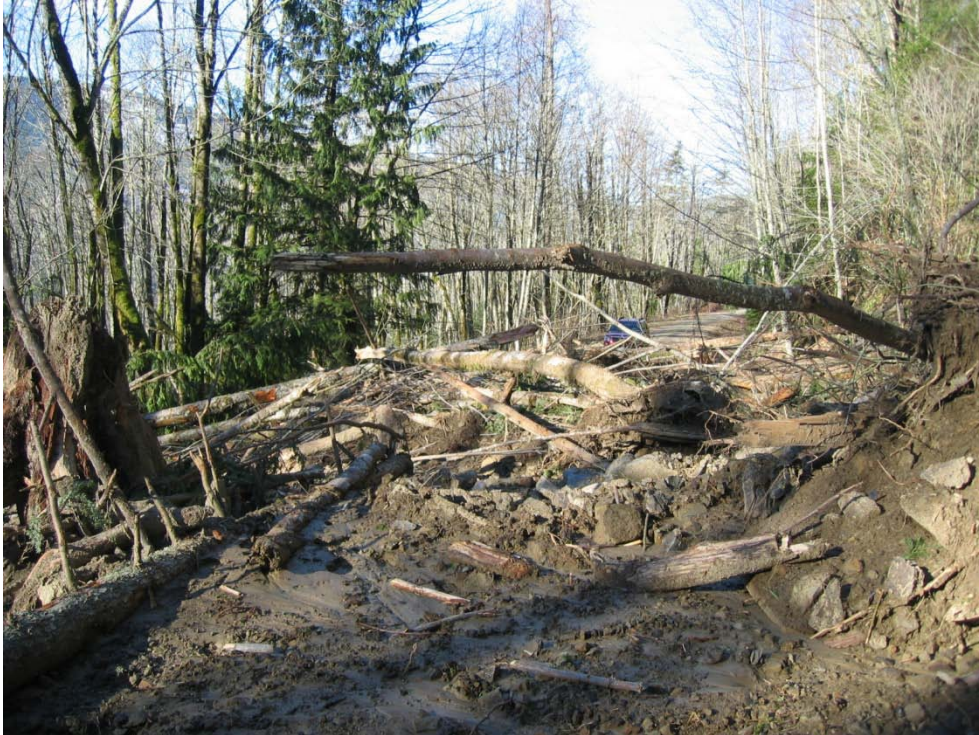
Figure 40 Debris from the Cliff Slide deposited on the CL-1000 Mainline Road. Photograph taken January 2009. View looking northwesterly. (Photo by M. Penney)
