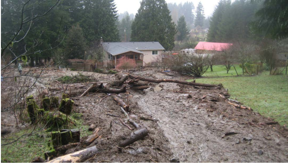
Figure 6 Debris flood across back of 3810 NR site. View looking northwest toward back of Fitch house. Photograph taken early January 2009. (Photo by D. Hooks)
