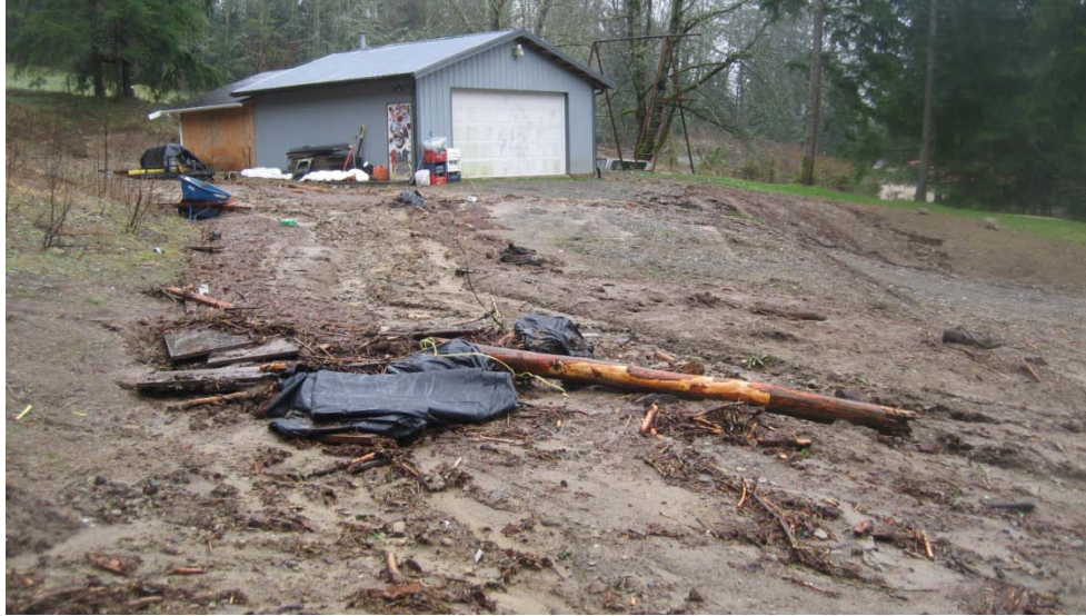
Figure 14 Garage/workshop at 3830 NR site. Debris hit far corner and then came toward viewer, some also came over slope in left of photograph. Photograph taken early January 2009. View looking south. (Photo by D. Hooks)
