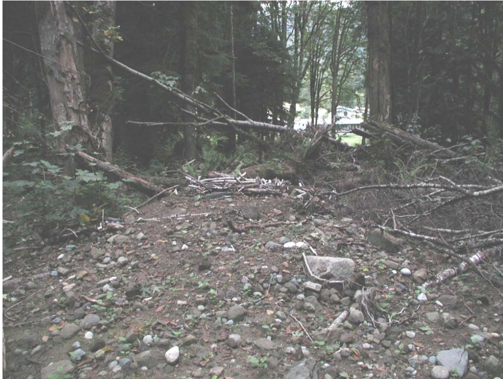
Figure 32 Debris deposited in trees at upper area of the alluvial fan. Kirkwood home in background through trees. Photograph taken in January 2009. View looking west. (Photo by M. Penney)
