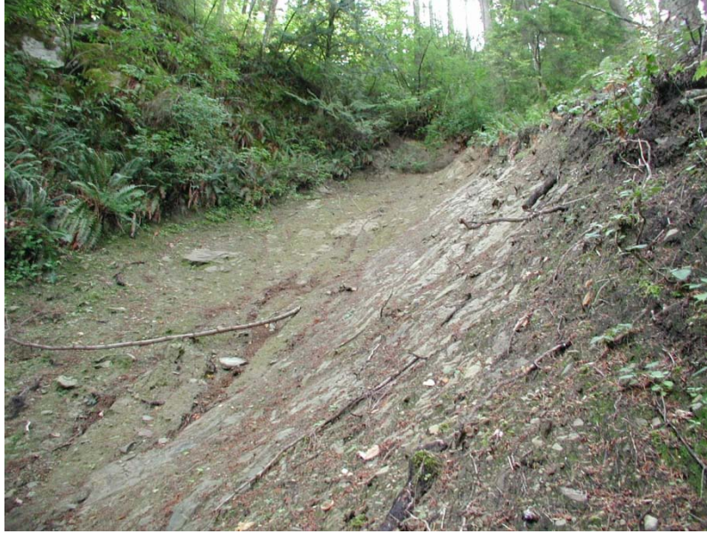
Figure 10 PI of the 3830 NR site (Malec). Photograph taken in Fall 2009. View looking east. (Photo by J. Coyle)
