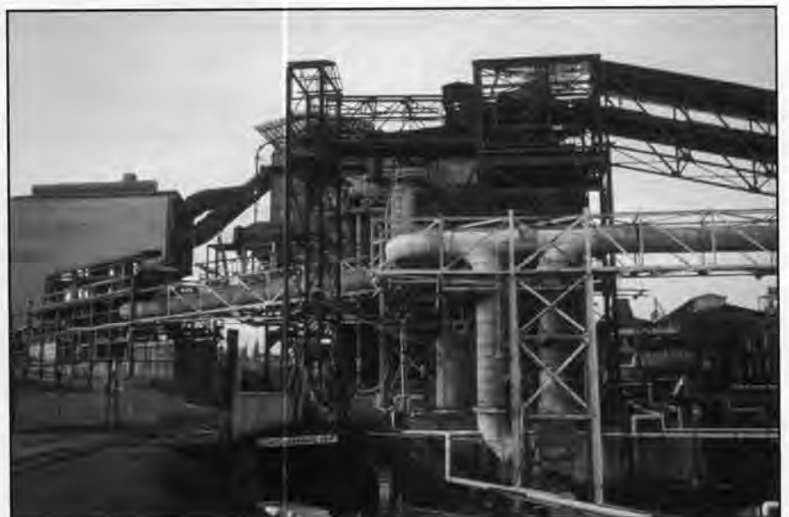
Figure 4. ASARCO smelter before demolition. Photo taken November 5, 1992.
