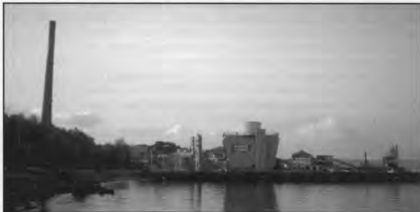
Figure 1. View of the ASARCO smelter to the west from Commencement Bay taken in 1992 before the smokestack was decommissioned and demolished (Jan. 17, 1993). The smokestack (on the left) was 572 ft 10 in. high. Built in 1917, for many years it was considered the tallest in the world.
