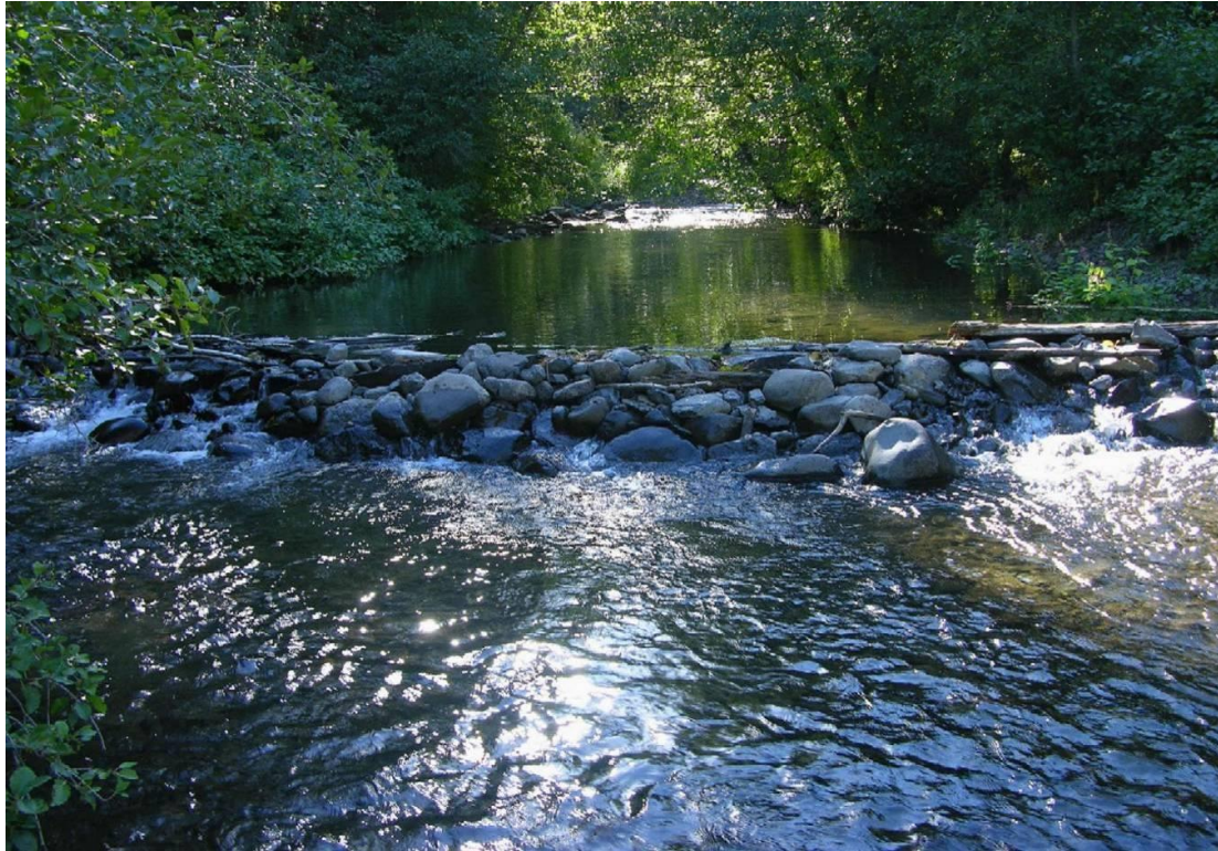
Figure 47. Recreational dam below the N.F./M.F. Ahtanum Cr. confluence.
