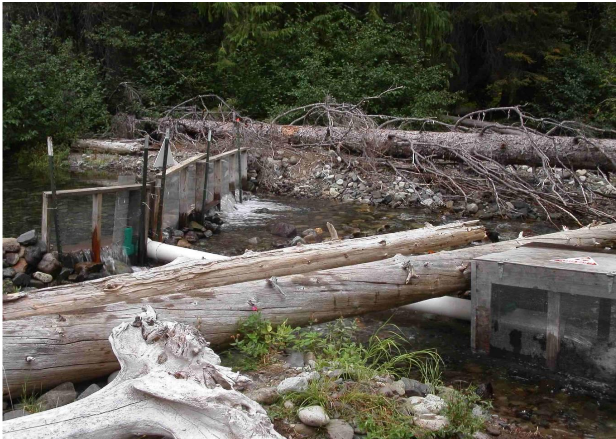
Figure 3. Union Creek “V” style panel weir and live box trap.
